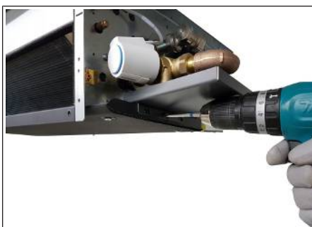
Fig. 73: Dismantle the valve condensation tray (ceiling model)
