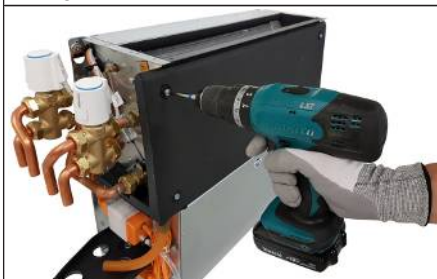
Fig. 71: Removing the main condensation tray (wall)
