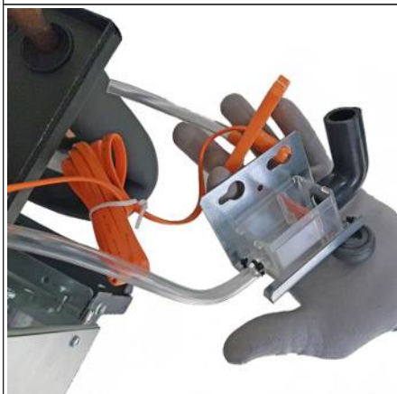
Fig. 76: Clean the float switch.
