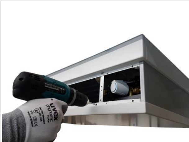
Fig. 9: Fix the casing with screws
