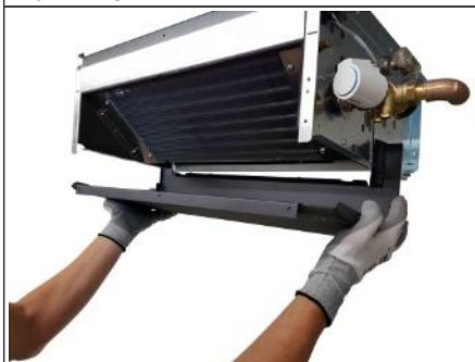
Fig. 70: Removing the main condensation tray (ceiling)
